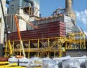
Atotal of approx. 200 t of steelwork was assembled for the supporting structure, maintenance platform and railings, and approx. 180 t of ducting with diameters of 3.00 m and 4.50 m was installed.
