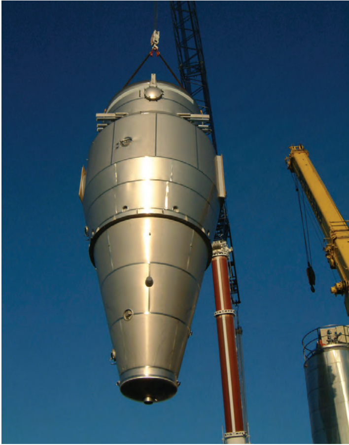
CIP filter for a spray dryer with a volume flow of 148.000 m 3 /h a.c.
