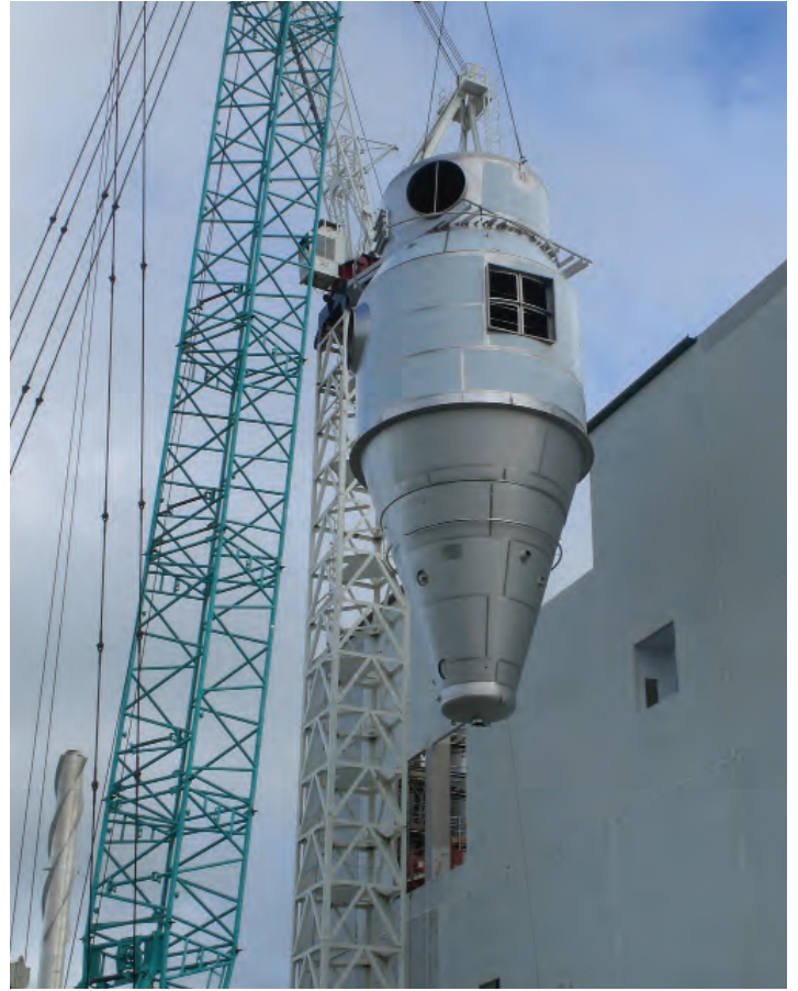
Assembly of the CIP filter for de-dusting of a spray dryer with a volume flow of 217.000 m 3 /h a.c
