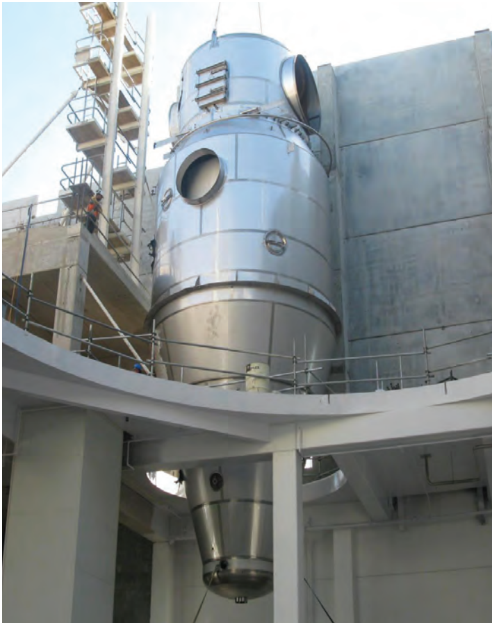
Assembly of the CIP filter for the world's largest spray dryer
